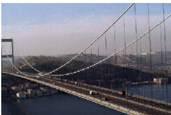
The Kinali – Sakarya Motorway (Second Bosphorus Bridge) in Turkey built with funding from OECF.
